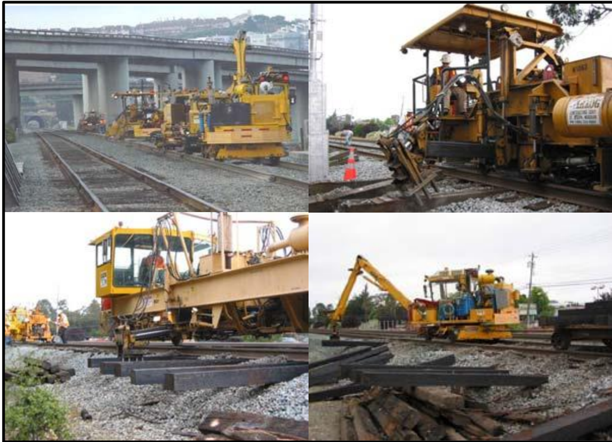
Figure 4: Crosstie Replacement Equipment
